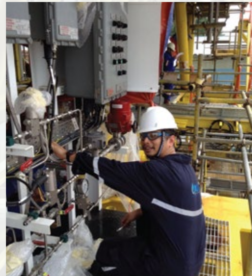
MAINTENANCE OF IGNITION SKID
